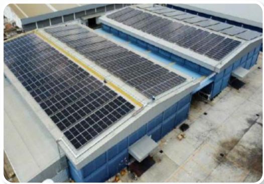
The roof of the original factory building.
